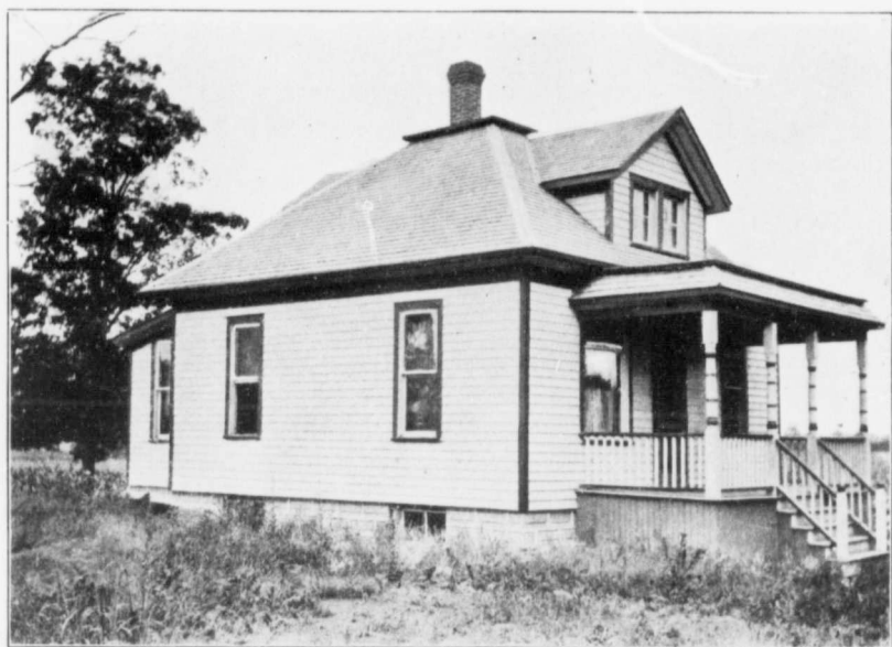
Harrow Experimental Station. Foreman's House.
