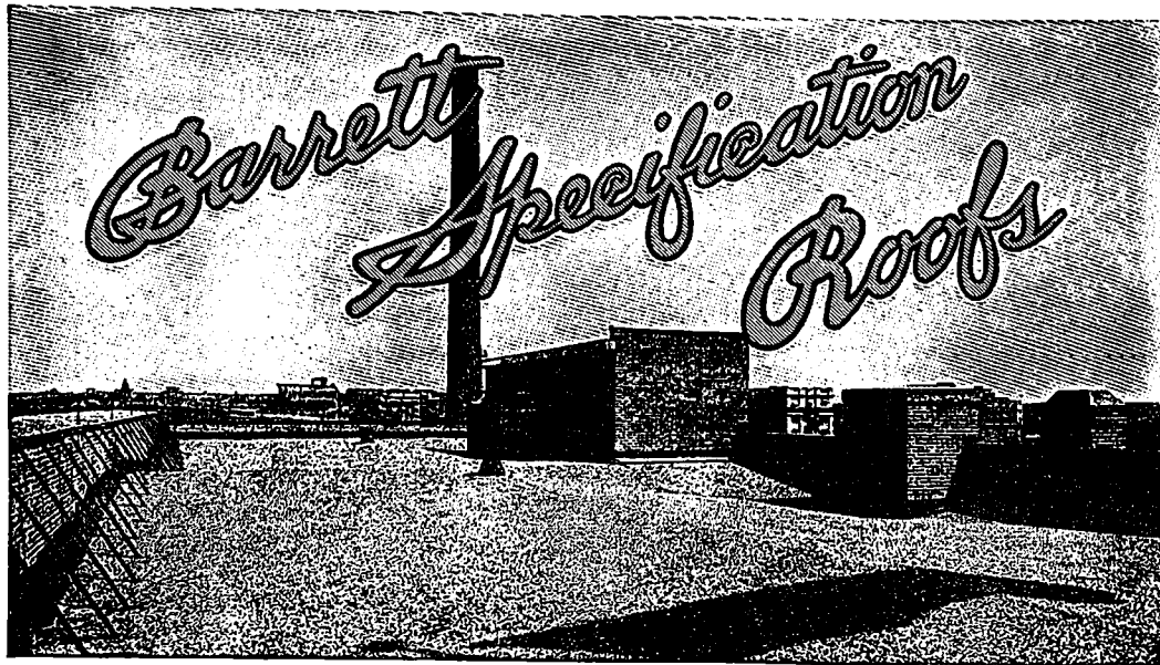
NORTHERN ELECTRIC COMPANY, CALGARY, ALBERTA.
