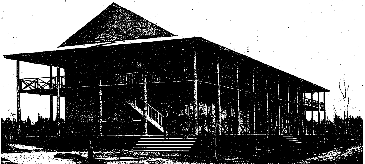
HEADQUARTERS OF THE R. F. C. AT CAMP HOARE, BORDEN.
