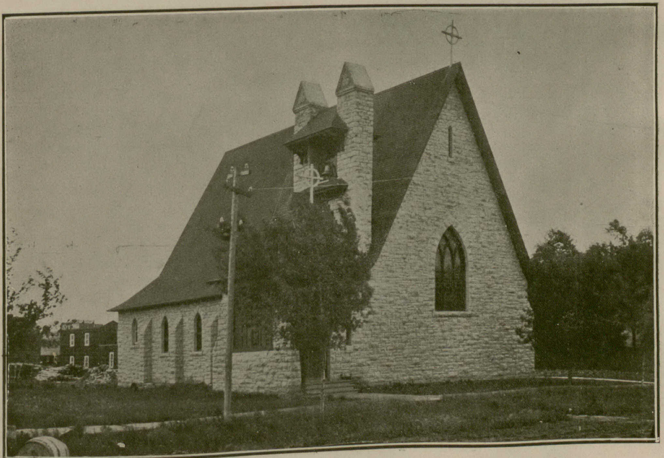
ST MARY'S CHURCH, PORTAGE LA PRAIRIE. H. S. GRIFFITHS, ARCHITECT, WINNIPEG.
