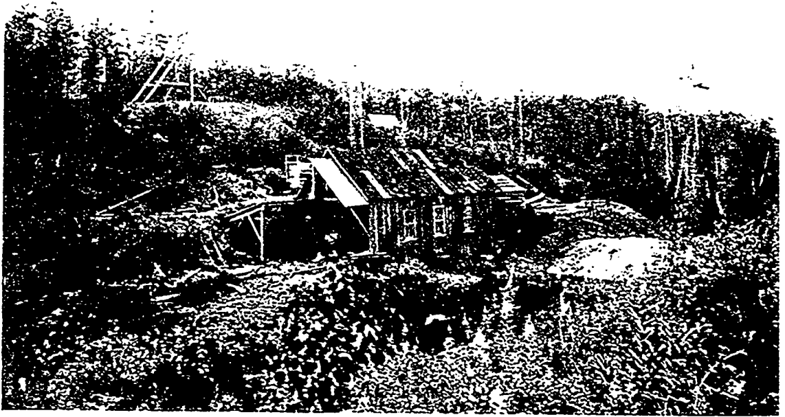
Surface Works at Lily May Mine, Rossland, B.C.
