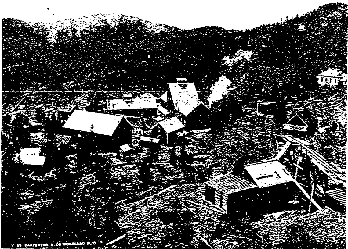
Surface Works of the LeRoi Mine, Rossland
