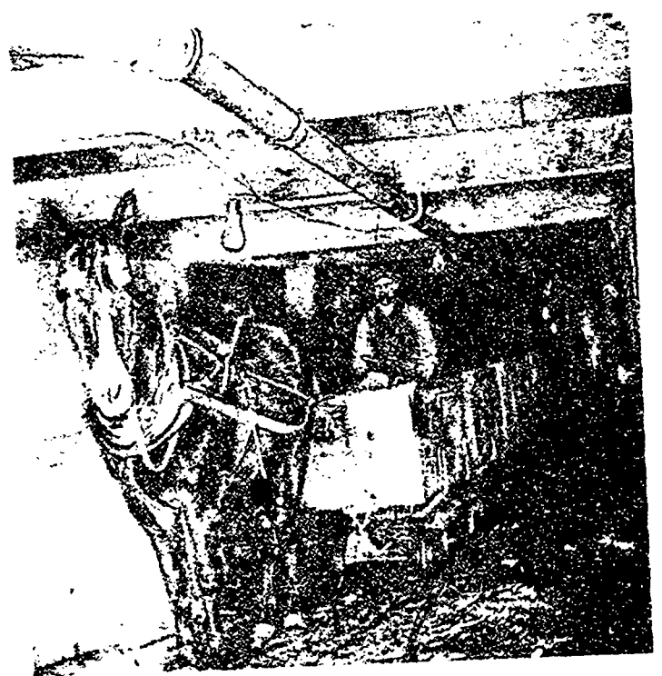
Mule Haulage, No. 5 Tunnel. Silver King Mine, Nelson, B.C.
