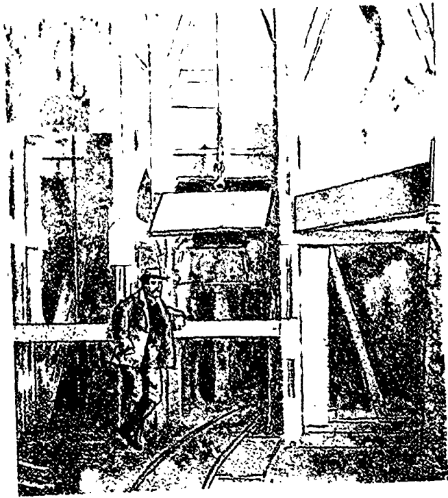
In No. 5 Tunnel, Main Shaft. Silver King Mine, Nelson:
