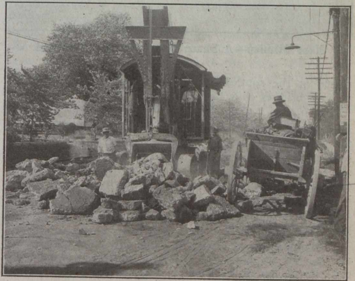
Tearing Up the Old Dolarway Road
