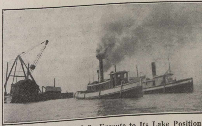
Fig. 9.—The Intake Crib, Enroute to Its Lake Position.
