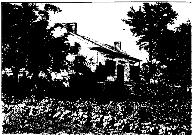
FIG. 1477.—MR. GEO. FISHER'S RESIDENCE.
