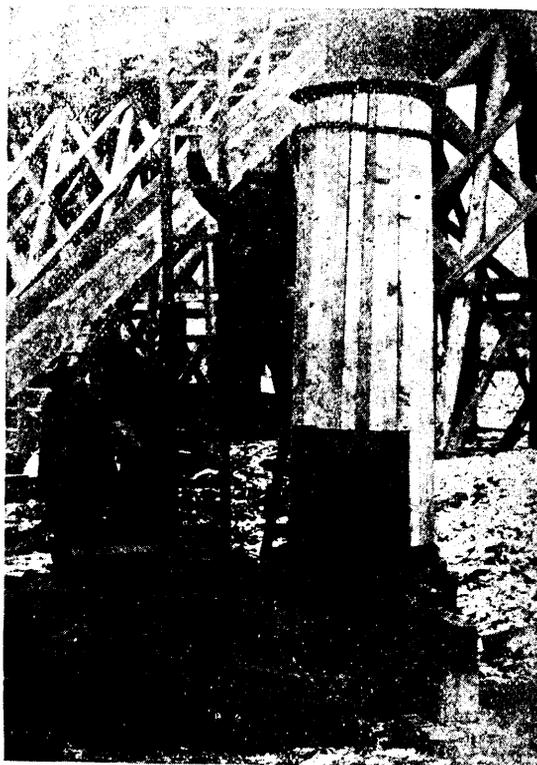
PREPARING THE WOOD PORTION OF THE ELEVATORS BEFORE PLACING THEM IN THE INCLINE.
