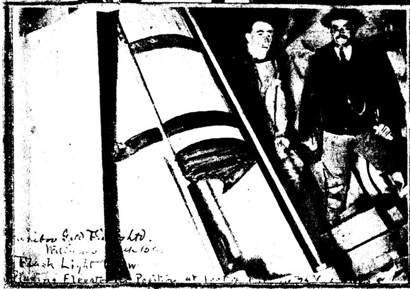
FLASH-LIGHT VIEW, PLACING ELEVATOR IN POSITION AT FOOT OF INCLINE 75 FEET BELOW SURFACE.
