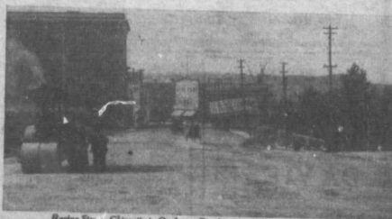
Rue de Ste-A, Chicoutimi, Quebec. Road constructed with "Tarvia-X"
