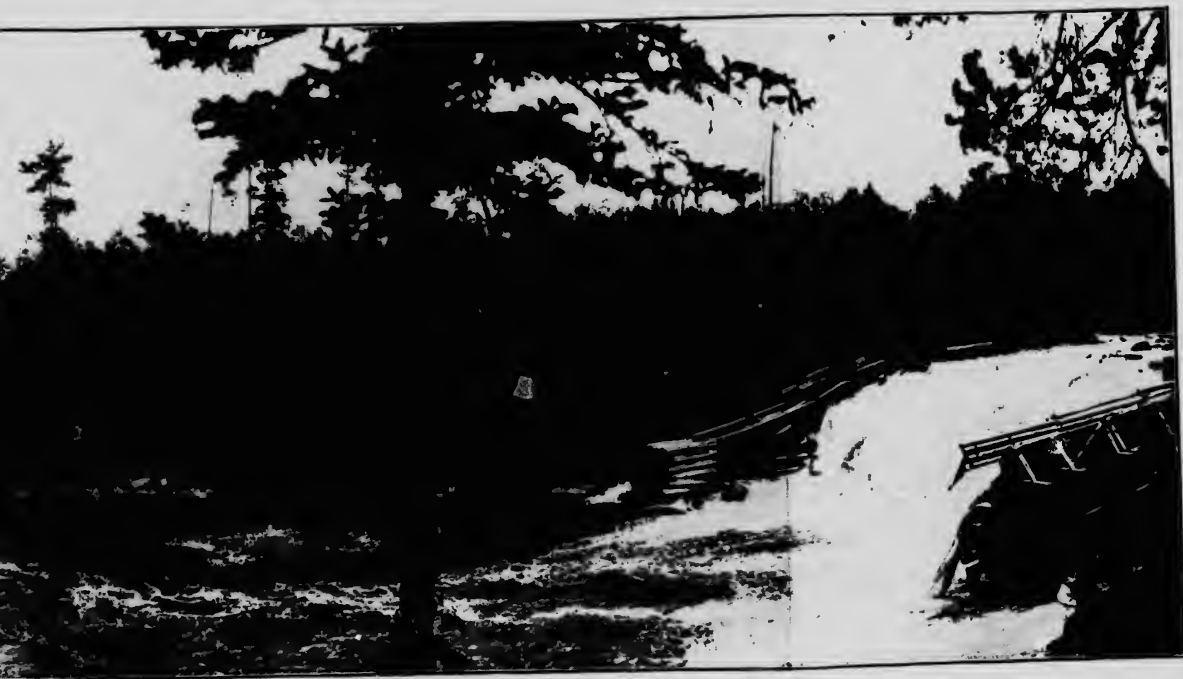
ls; water surface Deep River raised 23 feet—Canal passes behind side hill to left.
