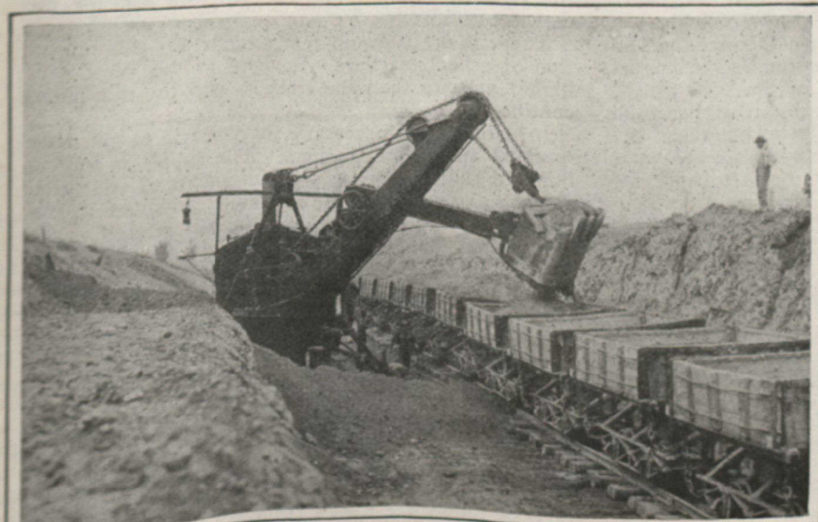
The steam shovel removing hundreds of tons a day, is a peculiarly American institution.
