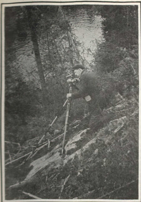
THE FIRST STEP IN CONSTRUCTION. A transit man on preliminary survey; the advance guard of an army of explorers.
