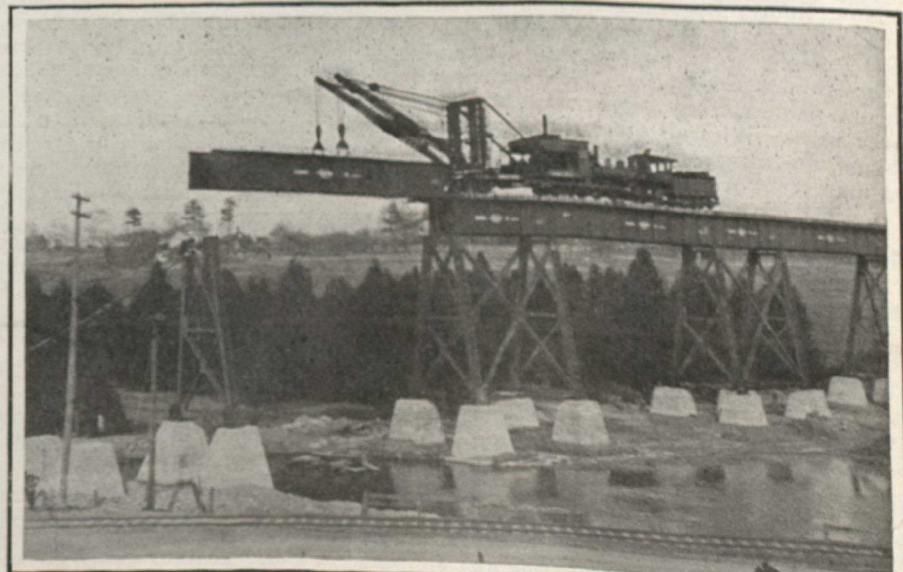
Swinging into place a steel beam of a big railway bridge.
