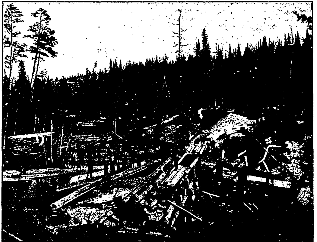
SCENES ON THE UPPER COULONGE—IMPROVEMENTS ON A CREEK. (In the early days less of this was done than at present, now the tendency is to shorten the haul by improving the streams.)
