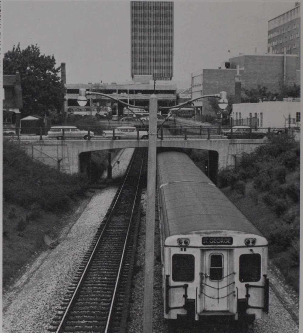
A train travels through an open-cut section of the Toronto subway system.
