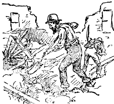
"I was helping dig out the cellar."
