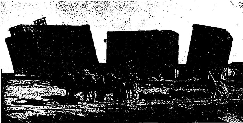
GRAIN WAREHOUSES IN TUNIS, AFRICA. A REMARKABLE PICTURE SHOWING TWO LARGE CONCRETE STRUCTURES THROWN 25 DEGREES OUT OF PLUMB, OWING TO ESCAPE OF QUICK SAND ON WHICH THEY WERE BUILT. BOTH WERE BROUGHT BACK TO A VERTICAL POSITION WITHOUT DEVELOPING A CRACK IN EITHER STRUCTURE. THIS WAS DONE BY LOADING SAND ON THEIR HIGH SIDE AND EXCAVATING UNDERNEATH.
