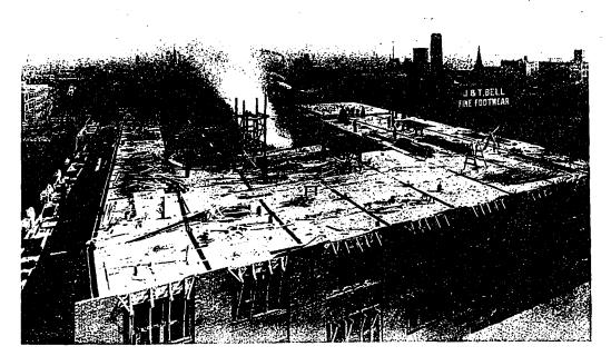
AMES-HOLDEN BUILDING, MONTREAL, SHOWING REINFORCED CONCRETE FLOOR WORK IN PROCESS OF CON-STRUCTION. IT WILL BE NOTED THAT THE FLOOR SUSTAINING EXTERIOR WALLS ARE CONSTRUCTED SIMULTANEOUSLY WITH THE CONCRETE FRAMEWORK OF THE BUILDING. ROSS& MACFARLANE, ARCHITECTS.
