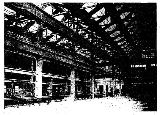
INTERIOR VIEW OF CONCRETE FACTORY, BUDAPEST. AN EXAMPLE OF THE ENTREMES TO WHICH THIS MATER-IAL IS EMPLOYED, THE SUPPORTING FRAME WORK AND ROOF TRUSS BEING ENTIRELY OF CONCRETE.
