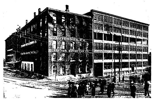
DAMAGED WAREHOUSE OF THE DAYTON MOTOR CAR COMPANY, DAYTON, OHIO, WHICH IS DEMONSTRATIVE OF THE FIRE-RESISTING PROPERTIES OF CONCRETE. THE FIRE STARTED ON THE FOURTH FLOOR OF THE CON-CRETE STRUCTURE ON THE RIGHT. WHERE IT BURNED ITSELF OUT. THE ADJOINING BUILDING TO WHICH THE FIRE WAS COMMUNICATED WAS COMPLETELY GUTTED.
