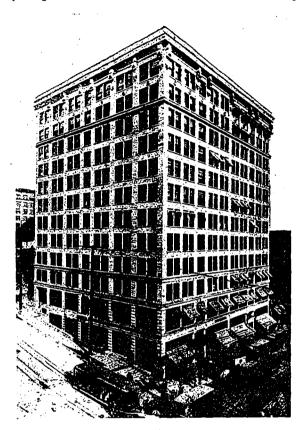
EMPIRE BUILDING, SEATTLE. Á. WARREN GOULD, ARCHI-TECT. ANOTHER EXAMPLE OF HIGH OFFICE BUILDING CONSTRUCTION OF WHICH THE ENTIRE FRAME-WORK IS OF REINFORCED CONCRETE CONSTRUCTION.
