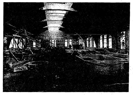
INTERIOR OF TELEPHONE BUILDING, SHANGHAI, CHINA, SHOWING ARCHED TRUSSES OF THE REINFORCED CONCRETE ROOF.
