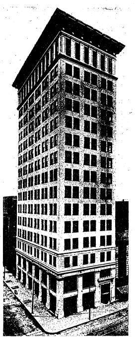
INCALLS BUILDING, CINCINNATI, OHIO, DESIGNED BY ELZNER AND ANDERSON. A SIXTEEN STOREY OF-FICE BUILDING OF REINFORCED CONCRETE SKELE-TON CONSTRUCTION, WHICH SHOWS HOW THIS MA-TERIAL IS BEGINNING TO COMPETE WITH STRUCTUR-AL STEEL IN THE SKYSCRAPER FIELD.
