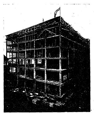
LYMAN SONS & COMPANY'S NEW BUILDING, MONTREAL. THIS BUILDING DEMONSTRATES THE POSSIBILITIES OF QUICK CONSTRUCTION'IN REINFORCED CONCRETE, THE FRAME WORK, INCLUDING ALL FLOORS AND THE ROOF, WAS COMPLETE TWO AND A HALF MONTHS AFTER EX-CAVATION. MITCHELL & CREIGHTON, ARCHITECTS.
