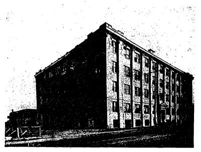
IMPERIAL TOBACCO COMPANY'S BUILDING, MONTREAL. A TYPICAL EXAMPLE OF AN ALL CONCRETE STRUCTURE. NOTE HOW SATISFACTORILY THE CONCRETE HAS ASSIMILATED THE ARCHITECTURAL LINES. MR. ROUERT FINDLAY, AR-CHITECT.
