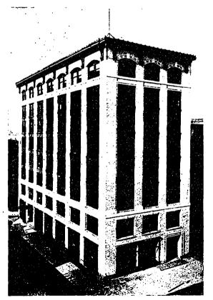
KAUN BUILDING, DETROIT, BUILT BY THE TRUSSED CON-CRETE STEEL COMPANY, IN ACCORDANCE TO THE SYS-TEM WHICH NAME IT BEARS. IT IS AN ALL CON-CRETE STRUCTURE WITH THE EXCEPTION OF THE EXTERIOR WALLS. MR. JULIUS KAHN, ARCHITECT.
