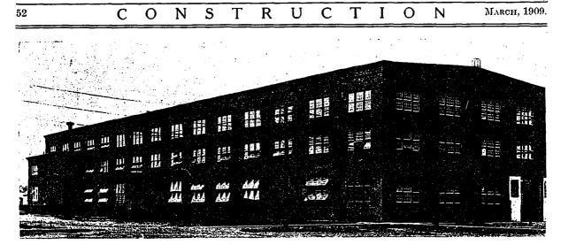
CANADIAN GENERAL ELECTRIC COMPANY'S TRANSFORMER HOUSE, PETERBORO. A STEEL FRAME STRUCTURE, WITH CONCRETE WALLS AND FLOORS.
