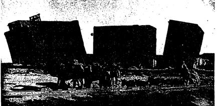
JRAIN WAREHOUSES IN TUNIS, AFRICA. A RE MARKABLE PICTURE SHOWING TWO LARGE CONCRETE STRUCTURES THROWN 25 DEGREES OUT OF PLUMB, OWING TO ESCAPE OF QUICK SAND ON WHICH THEY WERE BUILT. BOTH WERE BROUGHT BACK TO A VERTI-CAL POSITION WITHOUT DEVELOPING A CRACK IN EITHER STRUCTURE. THIS WAS DONE BY LOADING SAND ON THEIR HIGH SIDE AND EXCAVATING UNDERNEATH.
