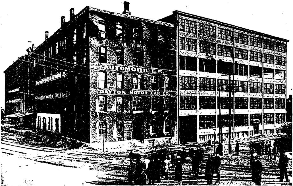
DAMAGED WAREHOUSE OF THE DAYTON MOTOR CAR COMPANY, DAYTON, OHIO, WHICH IS DEMONSTRATIVE OF THE FIRE-RESISTING PROPERTIES OF CONCRETE. THE FIRE STARTED ON THE FOURTH FLOOR OF THE CONCRETE STRUCTURE ON THE RIGHT, WHERE IT BURNED ITSELF OUT. THE ADJOINING BUILDING TO WHICH THE FIRE WAS COMMUNICATED WAS COMPLETELY GUTTED.
