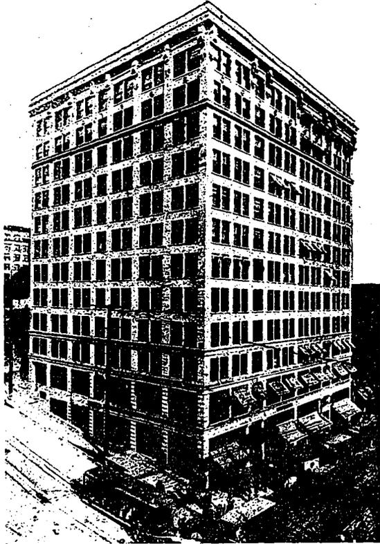
EMPIRE BUILDING, SEATTLE. A. WARREN GOULD, ARCHITECT. ANOTHER EXAMPLE OF HIGH OFFICE BUILDING CONSTRUCTION OF WHICH THE ENTIRE FRAMEWORK IS OF REINFORCED CONCRETE CONSTRUCTION.
