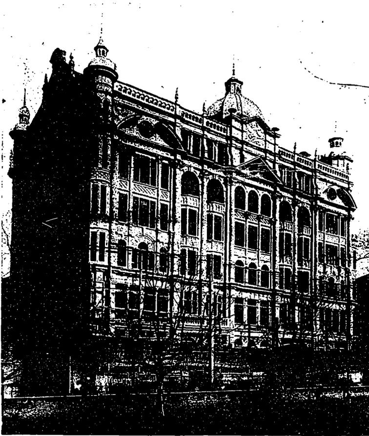
TELEPHONE BUILDING, SHANGHAI, CHINA. AN ELABORATELY DETAILED CONCRETE STRUCTURE, WHICH IS ESSENTIALLY A CARVED MONOLITH IN THAT THE EXTERIOR WAS ENTIRELY CUT BY HAND. MATHIEN & JARDIN, ARCHITECTS.
