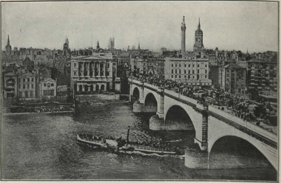
LONDON BRIDGE —The busiest and most crowded of all the bridges connects the City with the south of London. It was completed in 1831, at a cost of £2,000,000, under the superintendence of Sir John and George Rennie. In 1903 it was widened, being now 71 ft. broad instead of 54 ft., and a handsome granite balustrade substituted in place of the former solid sides. An extremely good view of the Tower Bridge can be obtained from here, while both interest and amusement can be gained by watching the various steamers which start in the summer for seaside resorts, etc.
