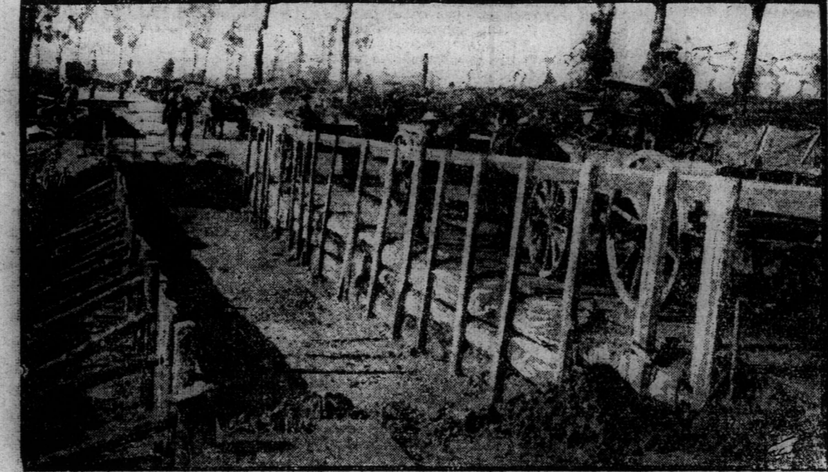
Near the Yser Canal.—Trees and supplies on their way to the battlefield.—Note the method employed of gradually building up the bridges to their proper level.
