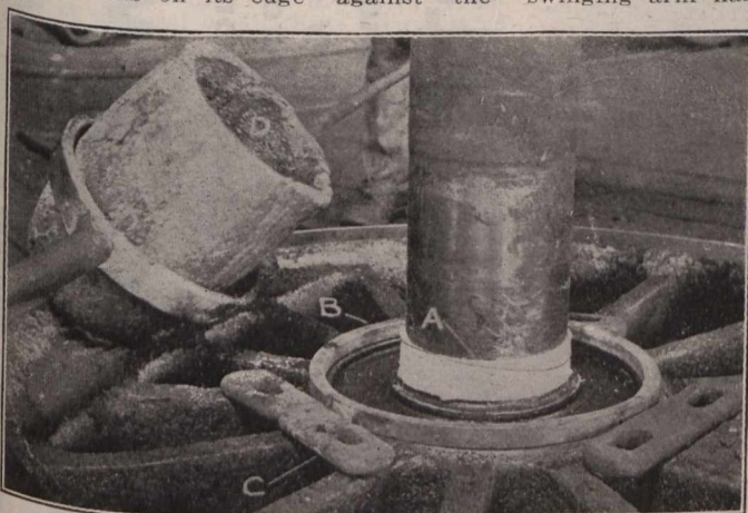
Fig. 1. Driving Wheels on End, ready for pouring.
