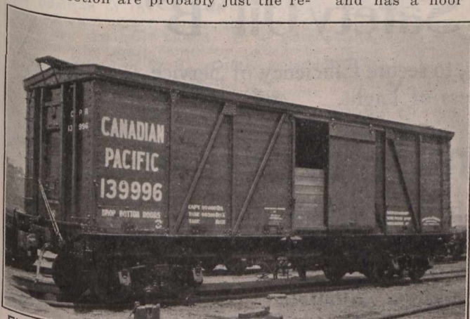
Fig. 4.—Exterior View of Completed Car with Dumping Doors open and Grain Door up.
