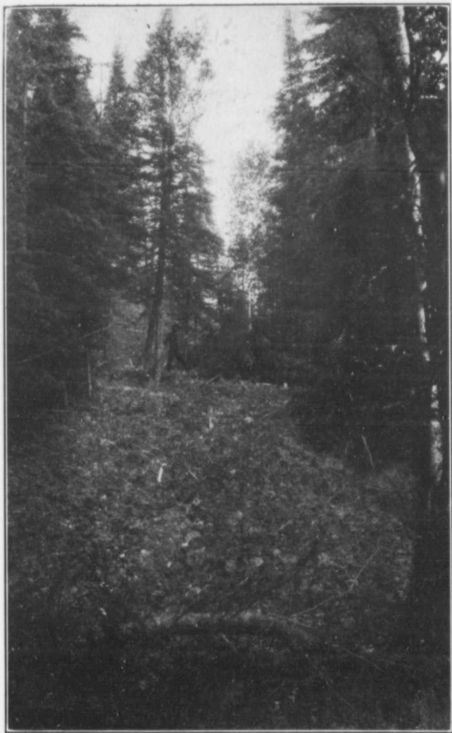
Beginning a Road.
