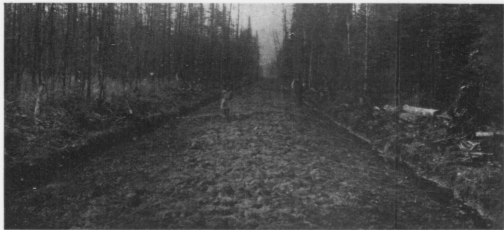
Newly Graded Road.
