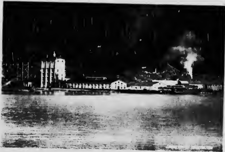
BRITISH COLUMBIA SULPHITE FIBRE CO'S PLANT, HOWE SOUND
