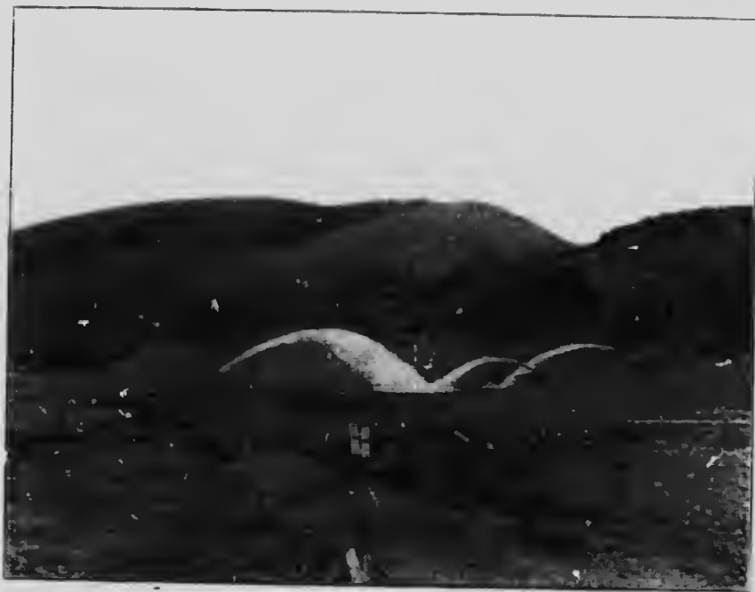
The hydraulic workings on the Saucerman property on the left bench of Thistle creek. Bedrock, which is here 50 to 60 feet above the creek opposite, is overlain by about 12 feet of gravel above which is 50 to 60 feet of muck and ice as shown in the high cut bank in the right of the view.
