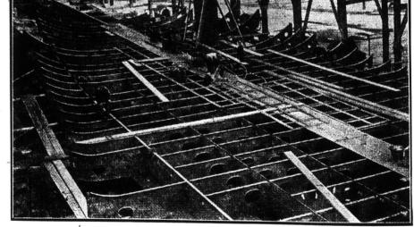
The floor of the ship : The official keel plate is the narrow strip leading away from the centre of the hulk
