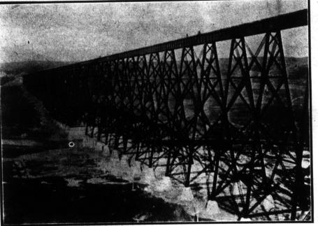
Battle River Bridge, Looking East. 180 ft. high, 2.770 ft. long. (Note man on bridge near Water Barrel)
