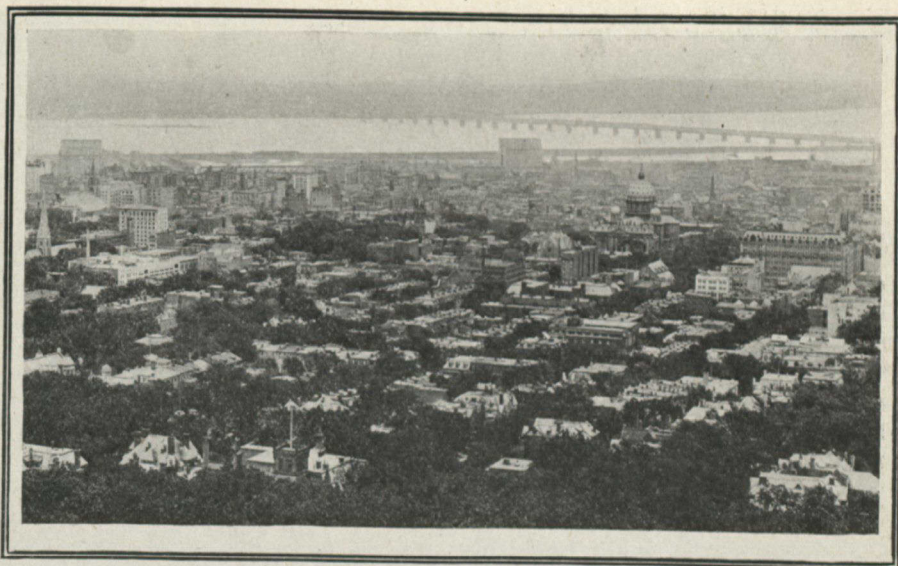
The City of Montreal, showing the River St. Lawrence, the Victoria Bridge, and the Dome of St. James's Cathedral
