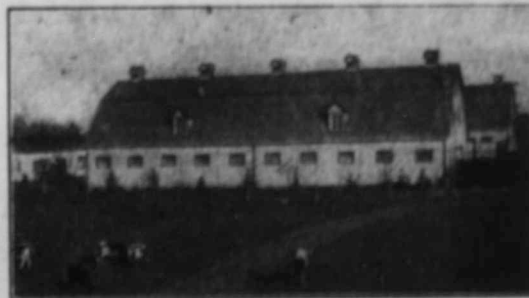
BUILDINGS ON THE BONNIE BRAES FARM
