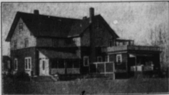
BUILDINGS ON THE BONNIE BRAES FARM
