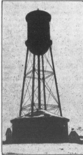
WATER TOWER, EAST TORONTO, ONT.
