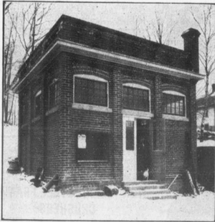
POWER HOUSE, EAST TORONTO, ONT.
