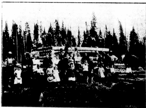
Building a Log House in New Ontario.
