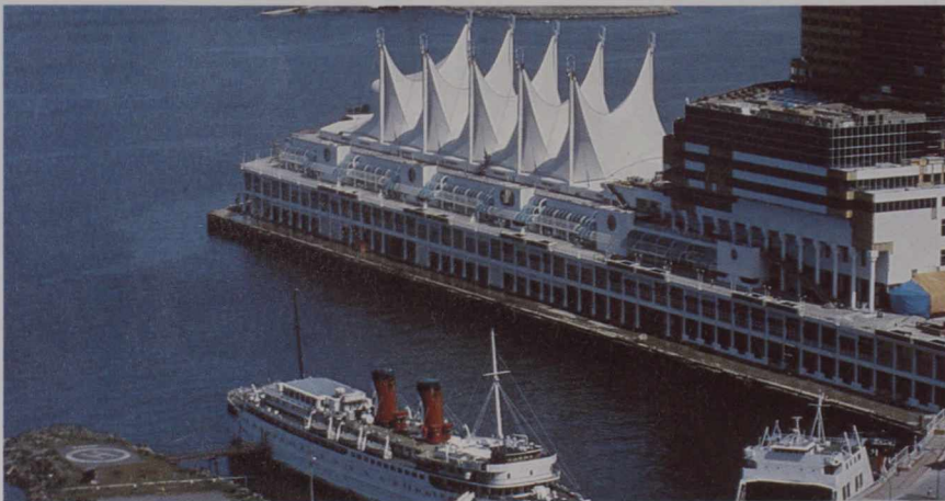
Canada Place — several buildings in one.
