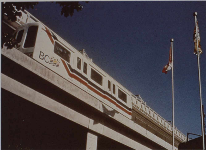
ALRT system operates automatically without driver or guard.
