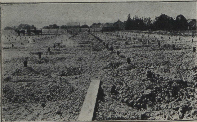
Filtering Bed, showing Sprinklers.
