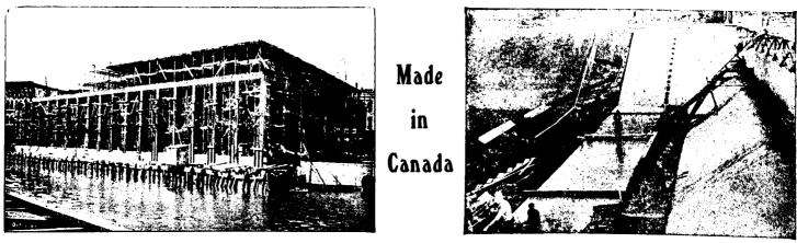
Bostwick-Brown Hardware Co. Building, Toledo, Ohlo. Walls and floor are 20 ft. below water level. "Medusa" Waterproofing used in basements
