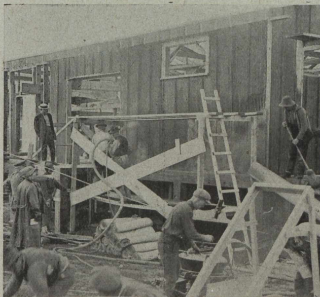
Construction of Camp Buildings.
