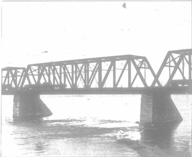
**VICTORIA BRIDGE, MONTREAL, QUEBEC.** Showing one span of new work. Masonry work under the water built with Thorold Cement in 1853-60. Messrs. Jackson, Peto, Brassey and Betts, London, Eng., contractors. Ross and Stephenson, engineers of the old bridge.
