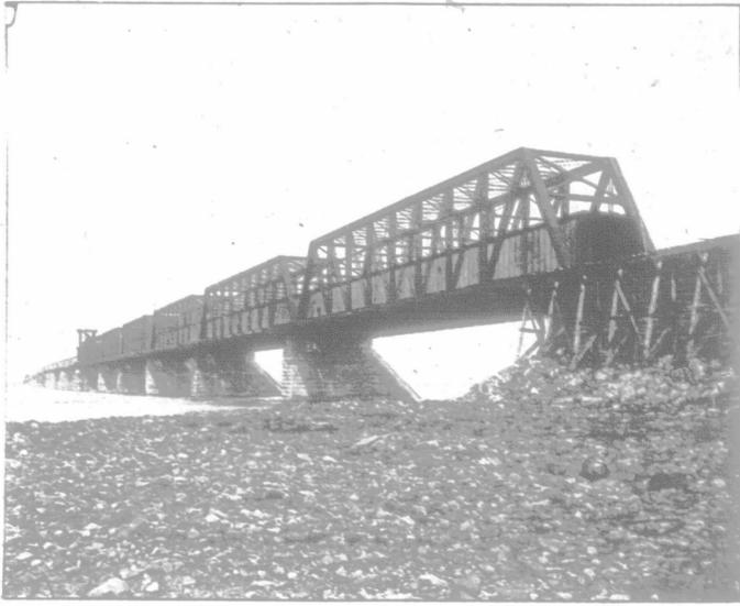
**VICTORIA BRIDGE, MONTREAL, QUEBEC.** Showing part of the old and new work. Masonry work under the water built with Thorold Cement in 1853-60. Messrs. Jackson, Peto, Brassey and Betts, London, Eng., contractors. Ross and Stephenson, engineers of the old bridge.
