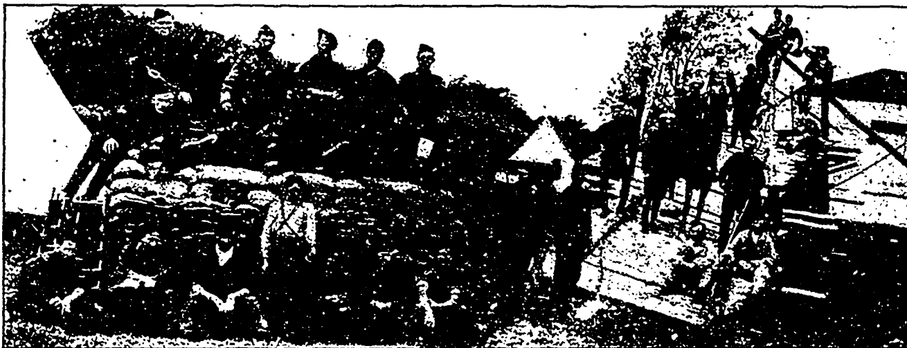
BREASTWORKS AND BRIDGE BUILT BY TORONTO ENGINEERS
