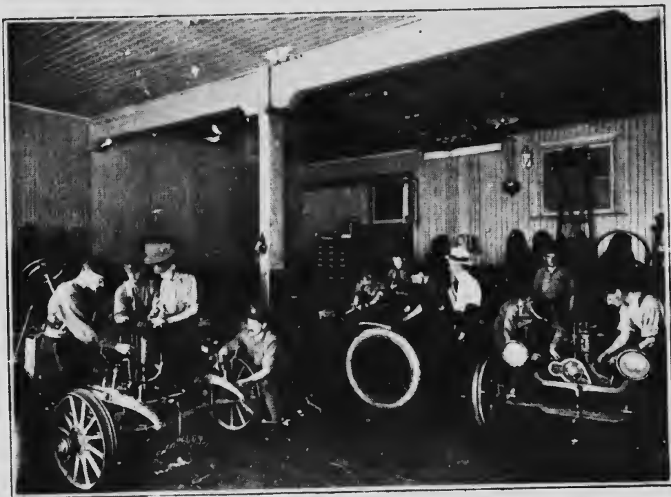
FIG. 101. Repair shop for automobiles. M. H. C., Canada.
