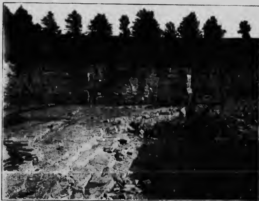
St. Marys quarries. Product used for building, and waste rock for road metal. Opening is 200 by 400 feet, and 20 feet deep. Perth County.
