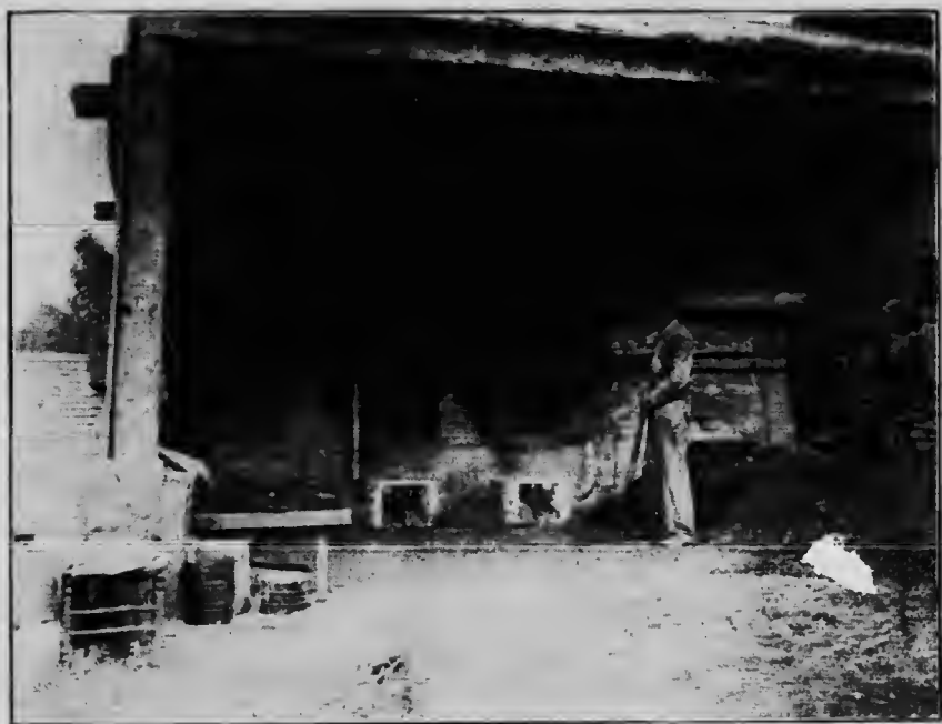
Lime kilns at Limehouse, showing double fire-door and forced-draught pipes. Halton County.
