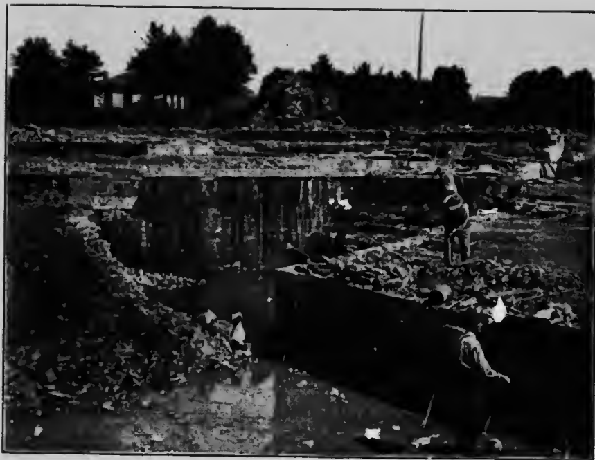
Elliott's limestone quarry, St. Mary's. Product used for building, and waste rock for road metal. Perth County.
