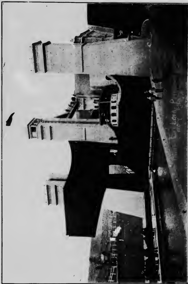
Hydraulic lift lock on Trent Canal, Peterborough, constructed mainly of cement; 26,000 barrels cement used in concrete work; substructure of lock said to be largest monolithic mass of concrete in the world.
