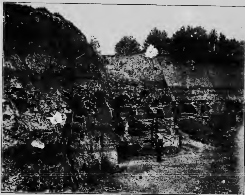
Selater's quarry, St. Marys. For lime burning only. Ten feet of earth and gravel overlying limestone, Perth County.
