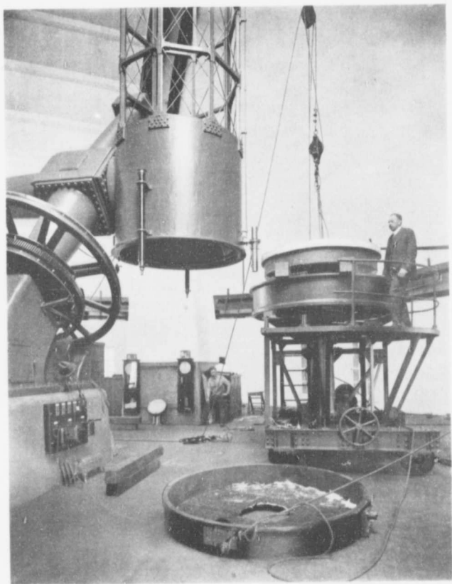
Fig. 4. Mirror resting on Cell on Silvering Car.
