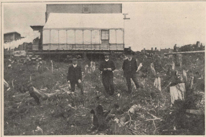
The way Houses are constructed at Prince Rupert. Board walls, tent roof. This is the Home of the Presbyterian Minister.
