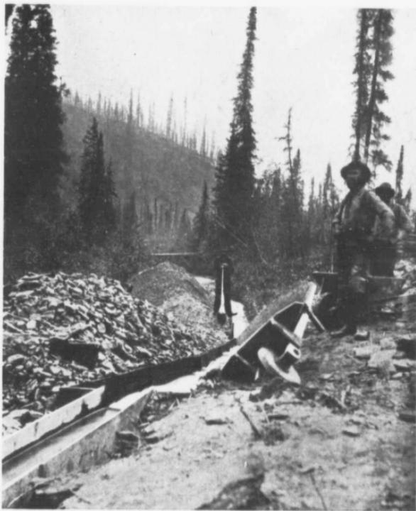
SLUICING ON BANANZA CREEK NO. 2 BELOW
