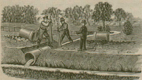
The bottom of the trench should be rounded out to fit as nearly as possible the curve
