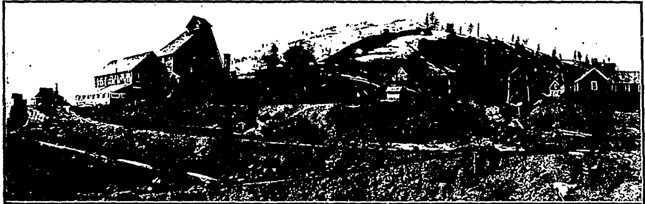
Head—Frame 85 ft. high, and Power House at Combination Shaft, about 1,500 ft. deep.
