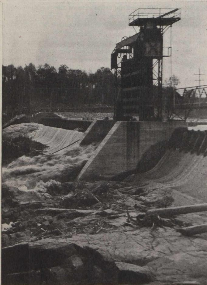
Fig. 10.—Close View of Open Sluice Gate.
