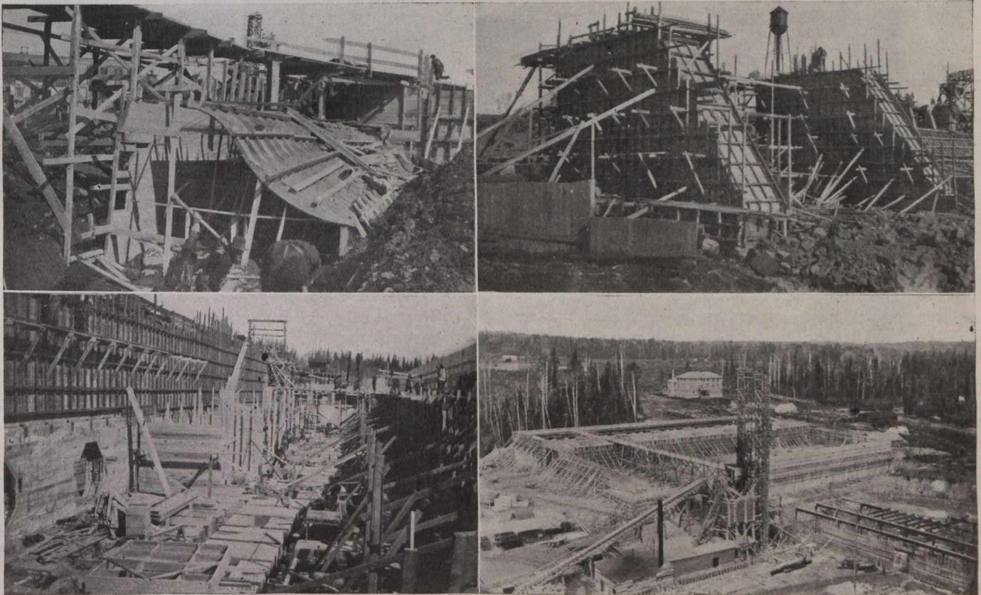
**Fig. 5.—Formwork Typical of Dam, Power House End of Dam. Breast Wall and Floor of Power House.**
