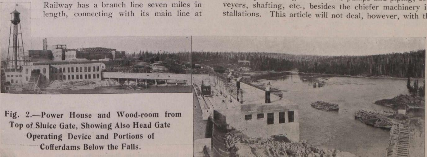
Fig. 2.—Power House and Wood-room from Top of Sluice Gate, Showing Also Head Gate Operating Device and Portions of Cofferdams Below the Falls.
