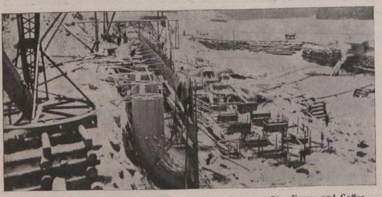
Fig. 7.—Power House Construction, Showing Draft Tube and Pier Forms and Cofferdam, Looking North.
