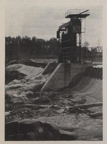
Fig. 10.-Close View of Open Sluice Gate.
