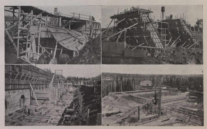
Fig. 5.-Formwork Typical of Dam, Power House and Mill Construction. Power House End of Dam. Breast Wall and Floor of Power House.
