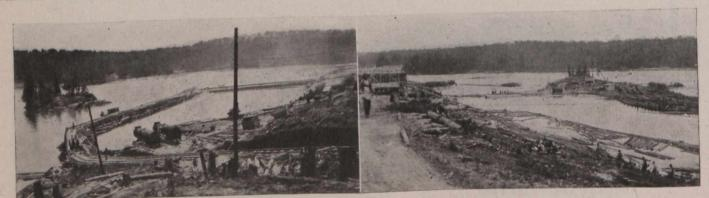
Fig. 4.-Cofferdams Above and Below the Falls Before Dewatering the Power House Site.
