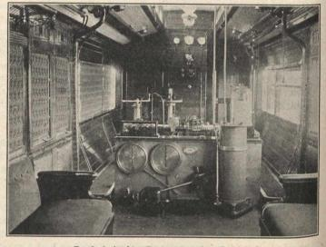
Back Interior Dynamometer Car.
