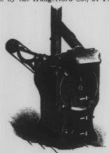
street, New York. The cut gives a very good idea of the appearance of the machine. Its dimensions are 8 feet high, 27 inches long and 20 inches wide. It is called the Portable XI. Roaster. and will roast coffee, peanuts, cocoaetc., and has just the capacity for a
