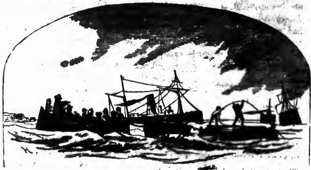
TAKING THE CABLE ASHORE.
