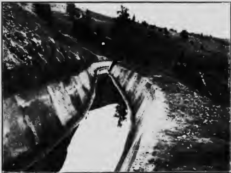
Fig. 25.—Concrete lined canal of Fruitlands Irrigation and Power Company, Kumloops, H. C.
