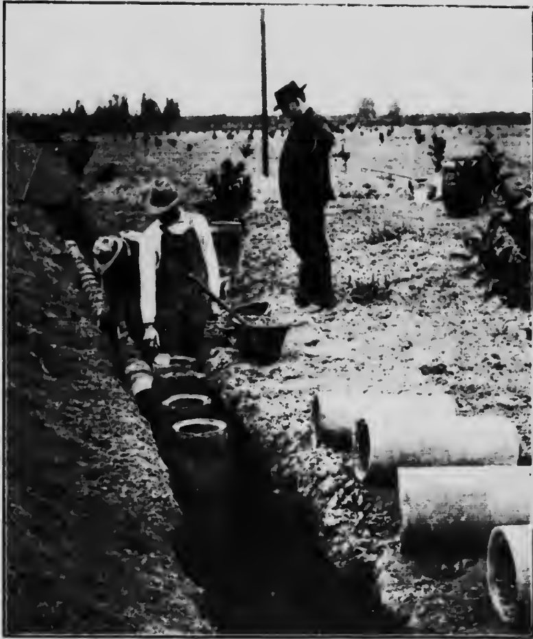
Fig. 30.—Method of laying and joining cement pipe.
