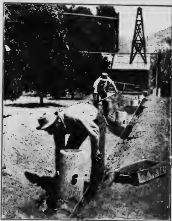
FIG. 69.—Construction of distributing stand pipes.
