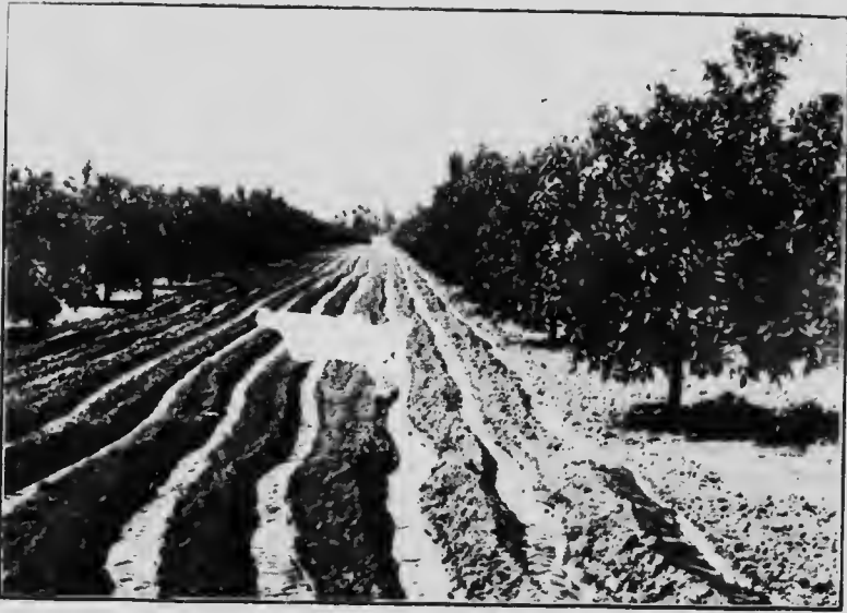
Fig. 61.—Distribution of water in furrows from concrete head flume.
