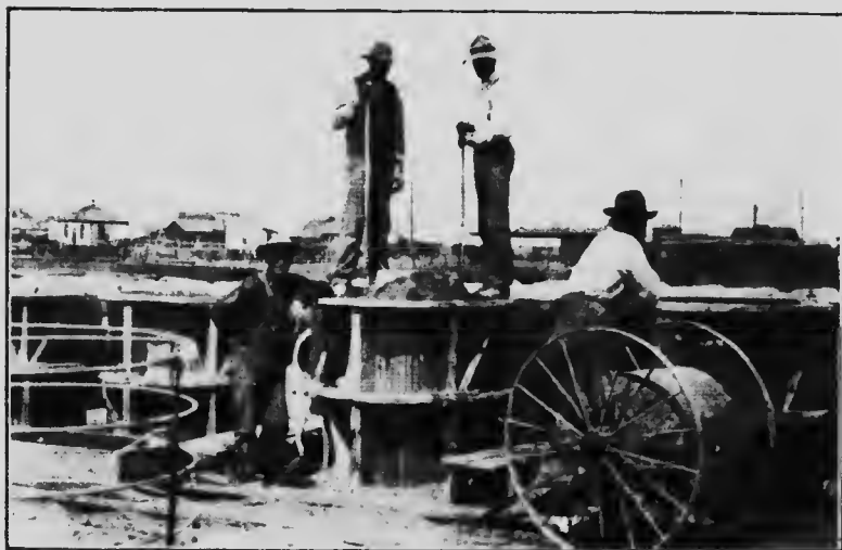
Fig. 43.—Placing concrete in moulds, Umatilla Project, Oregon.
