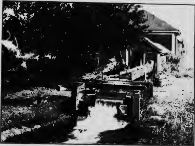
Fig. 8.—Rectangular weir box. (Courtesy of Irrigation Investigations Office, U. S. Dept. of Agr.)
