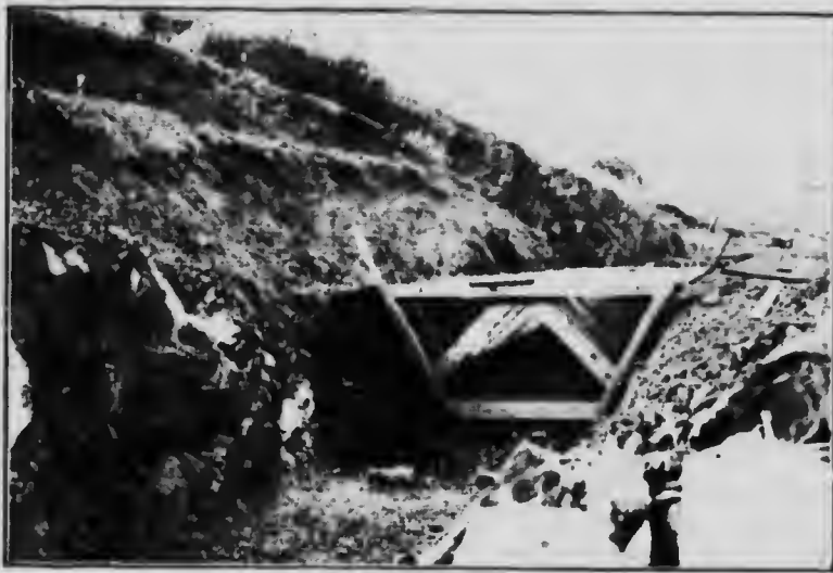
Fig. 27.—Method of using forms for backfilling to prepare canal for concrete lining, Fruitlands Irrigation System, Kamloops, B. C.
