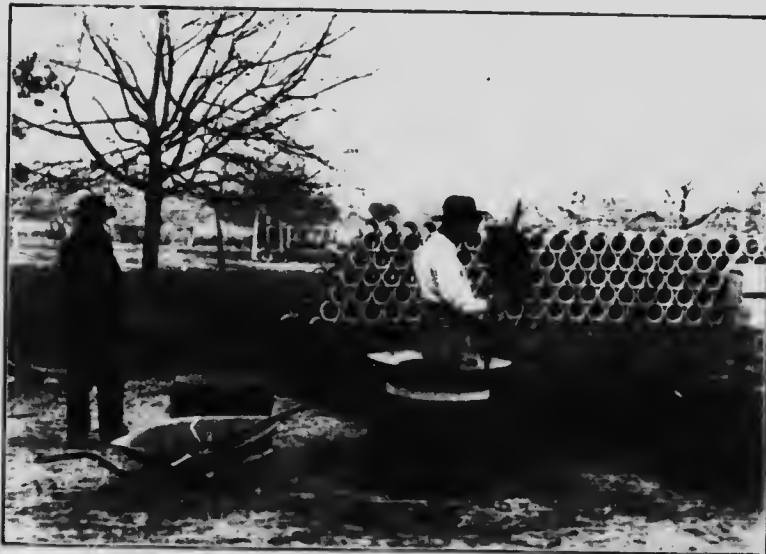
Fig. 37.—Process of tamping.
