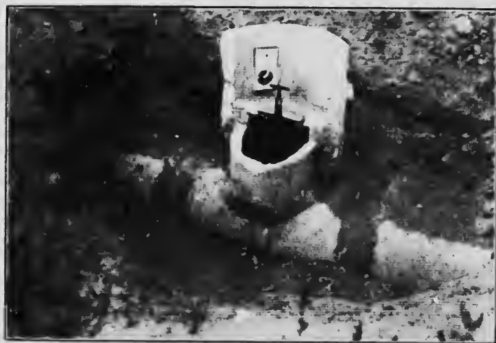
FIG. 70.—Distributing pressure stand pipe, type D.
