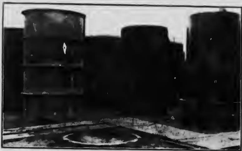
Fig. 10.—Molds for casting 48-inch reinforced concrete pipe, Umatilla Project, Oregon.
