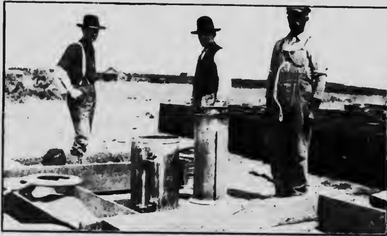
Fig. 36.—Moulds for casting hand-tamped pipe, showing inside core in position.
