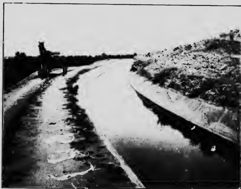
FIG. 34.—Concrete lined canal, Gage Canal Company, Riverside, Cal.
