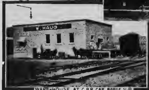
WARE-HOUSE AT C.P.R. CAR BARGE SLIP
