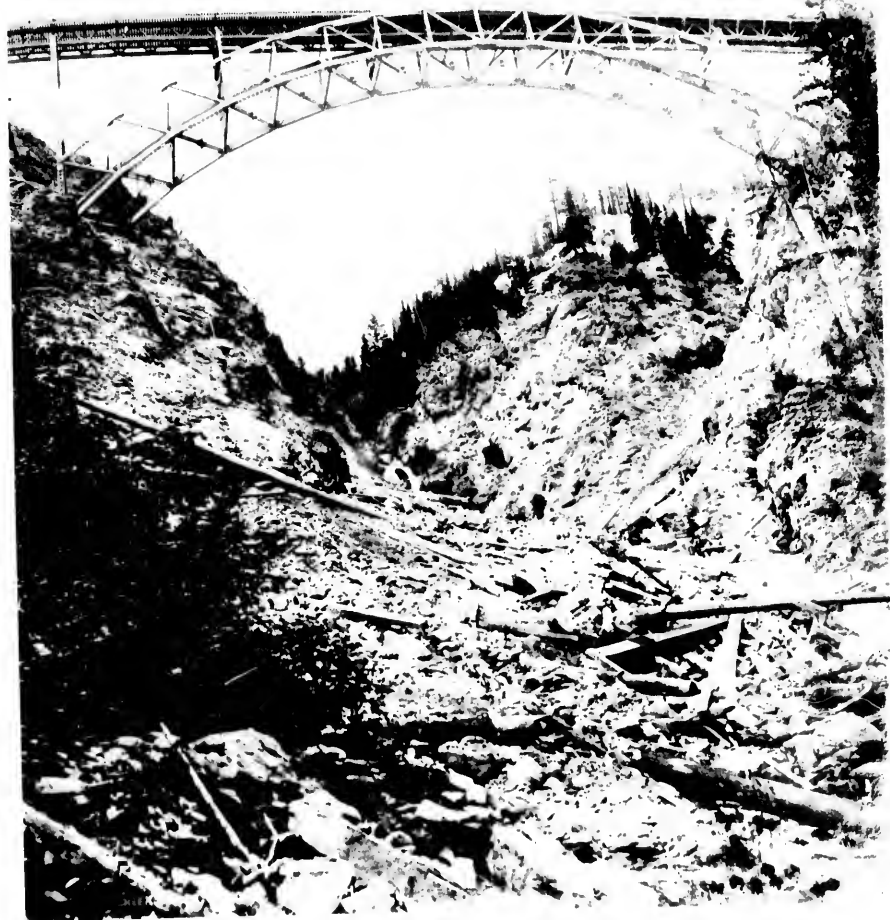
STONEY CREEK BRIDGE 296 Feet High.
