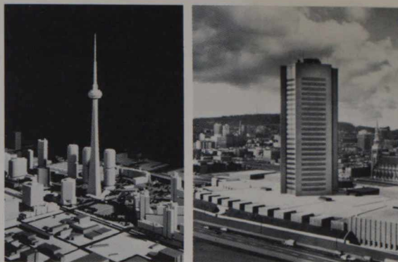
Left, CBC's Toronto Transmission Supertower, right, Place de Radio-Canada in Montreal.
